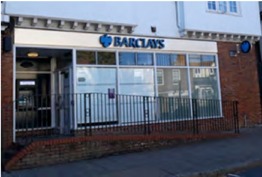
Figure 48 - Both the ramp and shopfront make for an unacceptable impact on the building and streetscene
