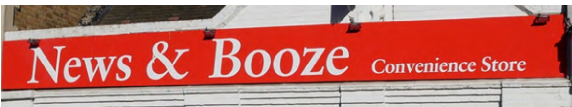
d) A plastic fascia board that is overly bright with large lettering and external lights that overpowers this building.
