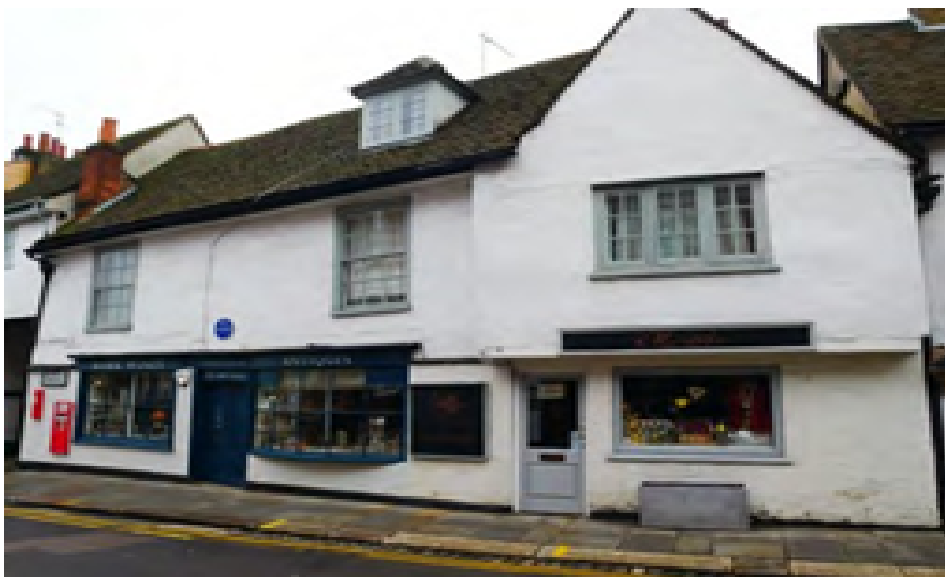
Figure 14: Signage respecting the medieval buildings.
