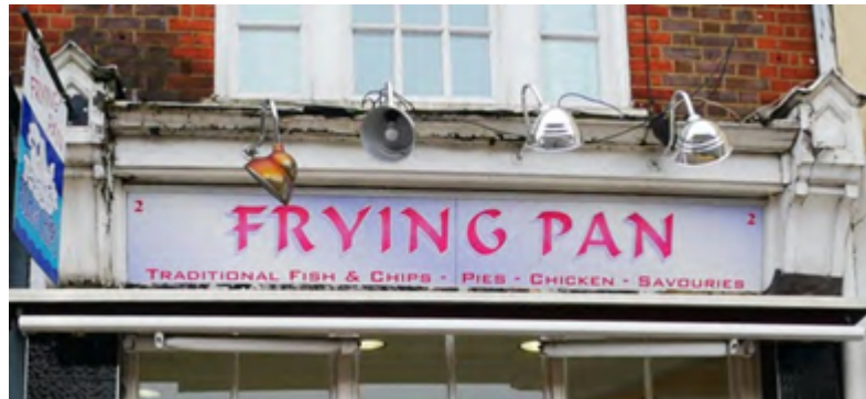
Figure 40 – Unnecessarily extensive lighting.
