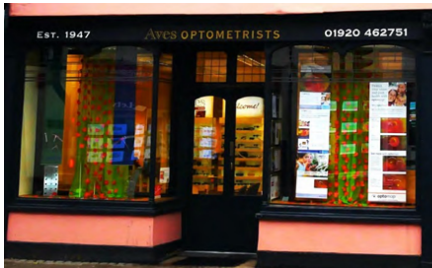
Figure 36- Appropriately scaled lettering to height of fascia.
