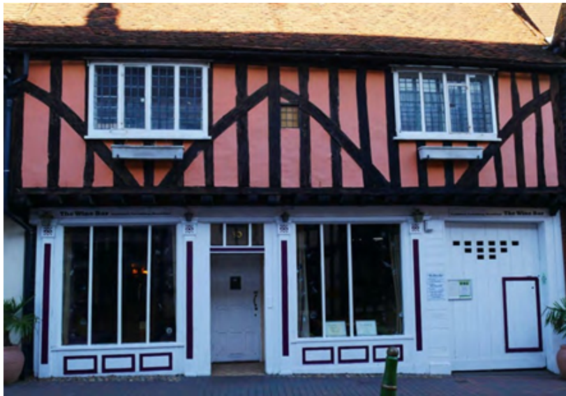
Figure 1 – Formerly a house but adapted to provide a double fronted shop to the ground floor.
