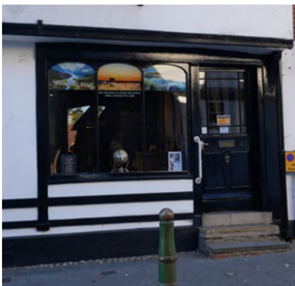
Figure 15 – An early 18th century shopfront inserted into a medieval building with simple detailing (Buntingford).
