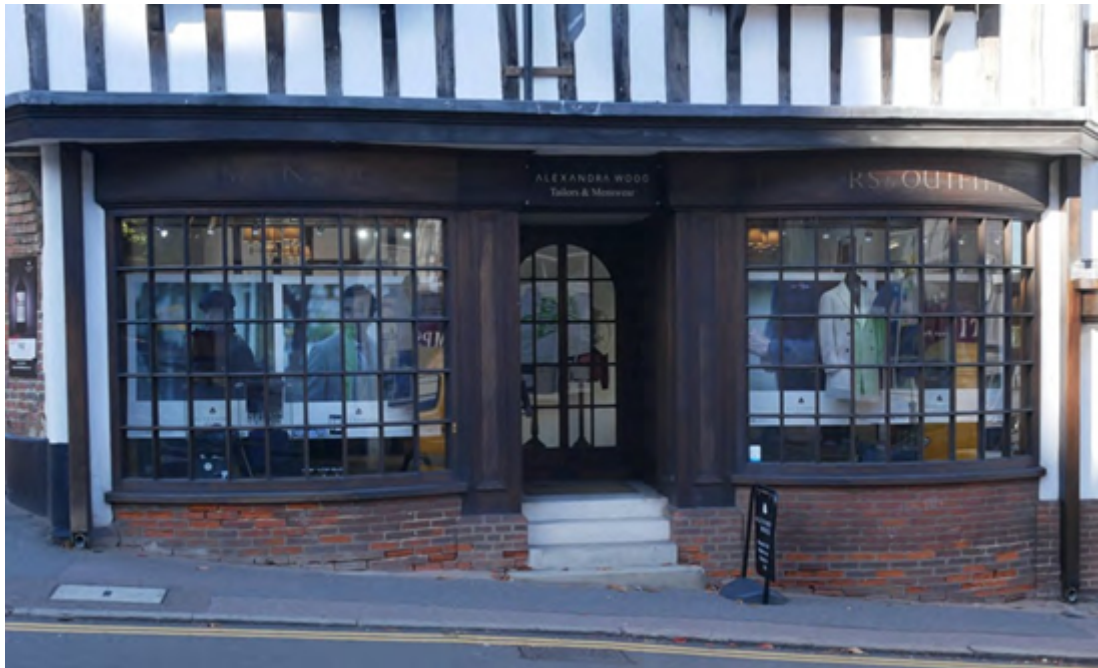
Figure 9 – a 15th century timber-framed house converted to retail use on the ground floor. The shopfront dates from the early 20th century and is of an appropriate design.
