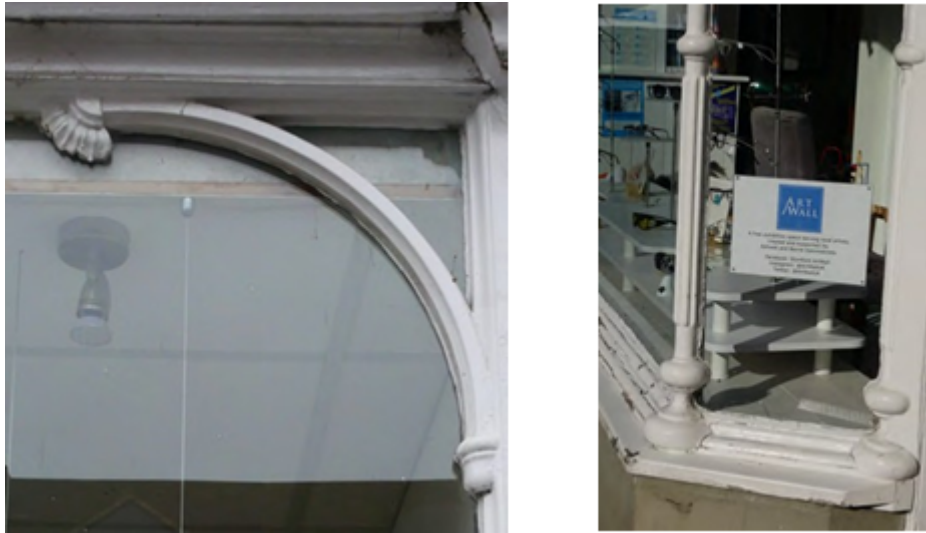
Figure 34 - An interesting Edwardian decorative glazing bar and a moulded mullion from the late-19th century.
