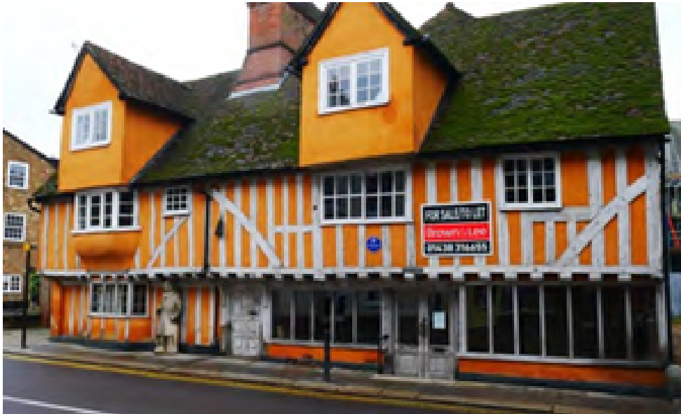
Figure 13 – The 15th century jettied, timber-framed building, St. Nicholas Hall or Verger's House accommodating retail.
