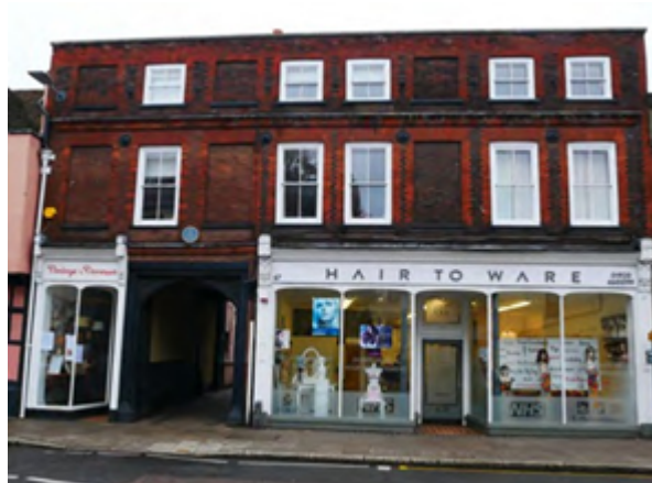
Figure 7 - A late 19th/early 20th century shopfront with traditional elements.
